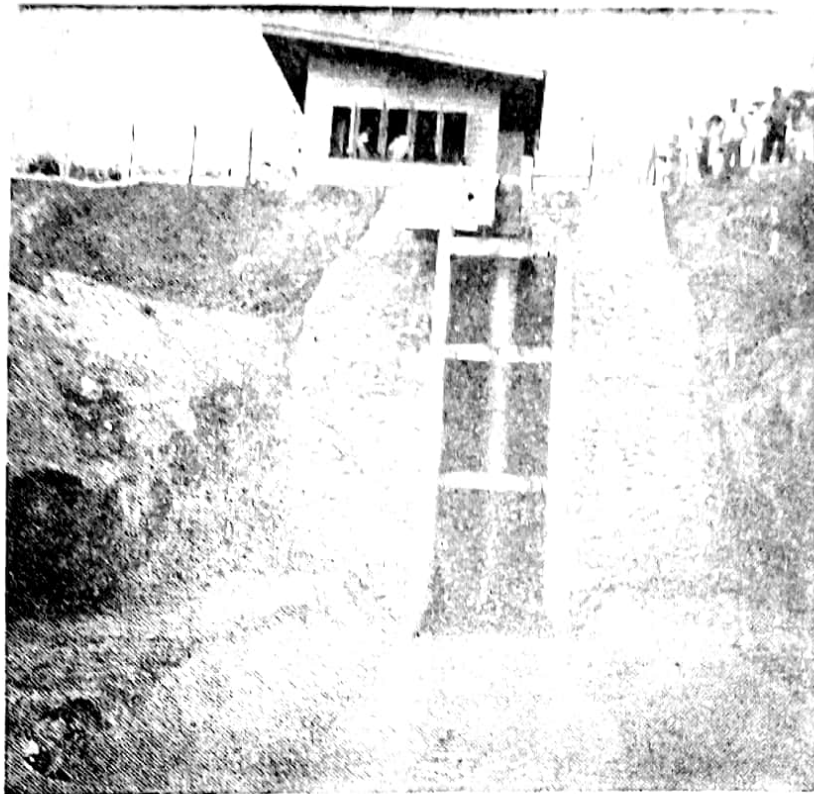
A high lift 16-inch pump installed in Magsalisi, Jaen, N.E., to irrigate 200 hectares of riceland.
